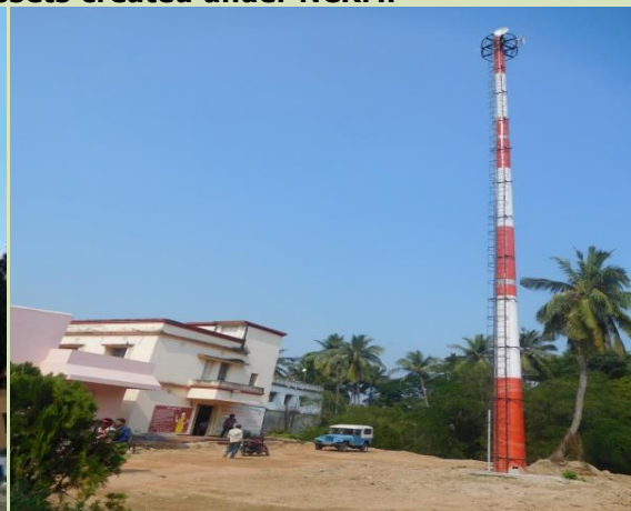
EWDS (Alert Siren) at Basudevpur, Odisha
